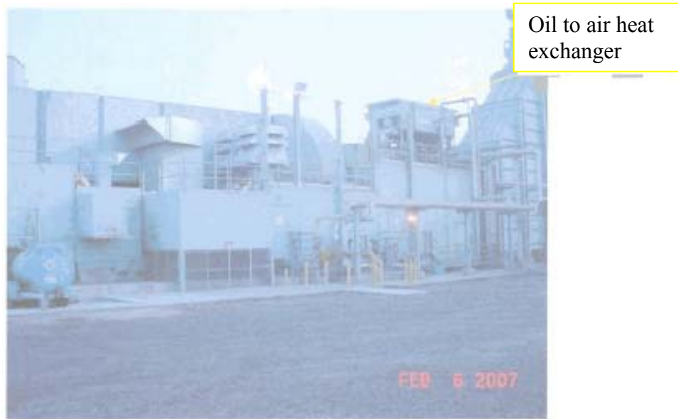
View of the Combustion Turbine package from the southwest. Shows the start pack, generator inlet air filters, turbine inlet air filter (evaporative cooling tower)
