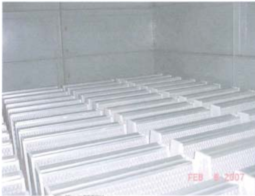
View of the generator enclosure from within the air inlet filter housing with the panel at the gearbox end removed.
