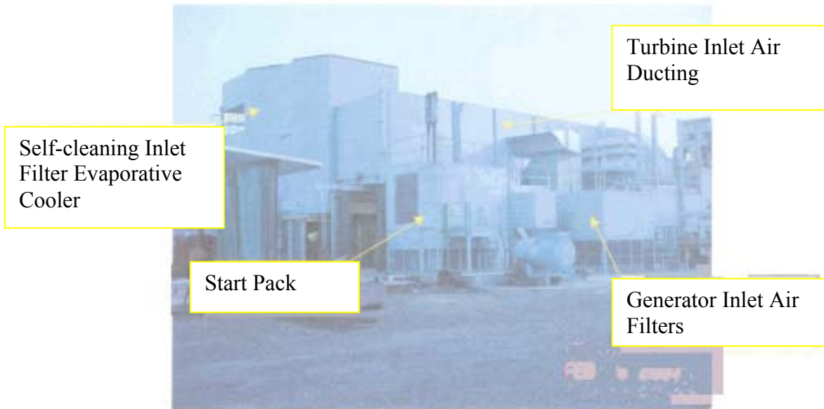
View of the Combustion Turbine package from the southwest. Shows the start pack, generator inlet air filters, turbine inlet air filter (evaporative cooling tower)
